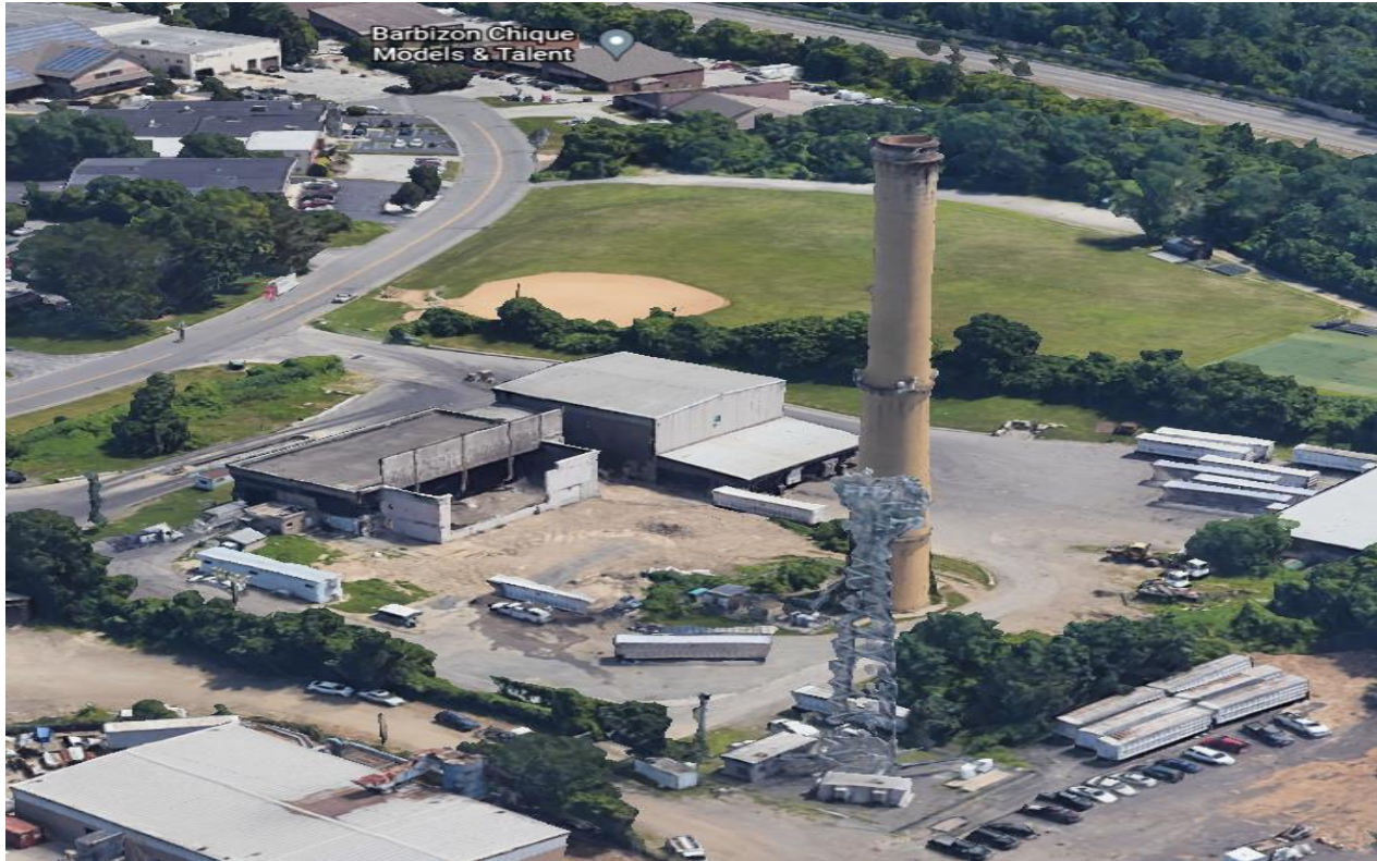
Transfer Station #3 (Broomall)
