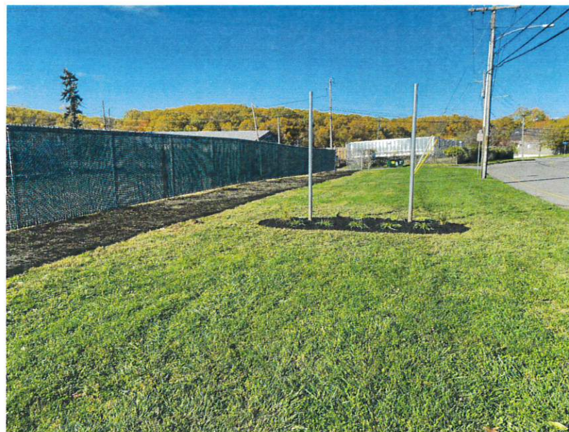
New Fence with New Signposts
